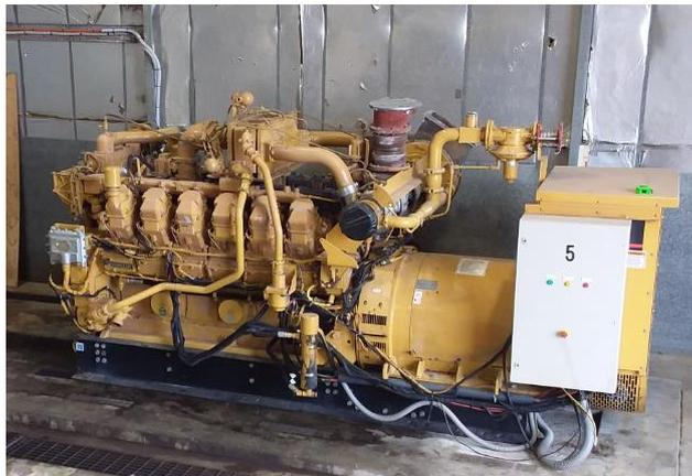
*Second CAT 770kW engine in position for installation.*
